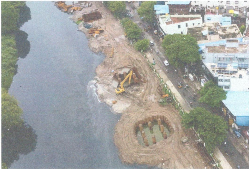
Excavation P93 @ Km 3+590
