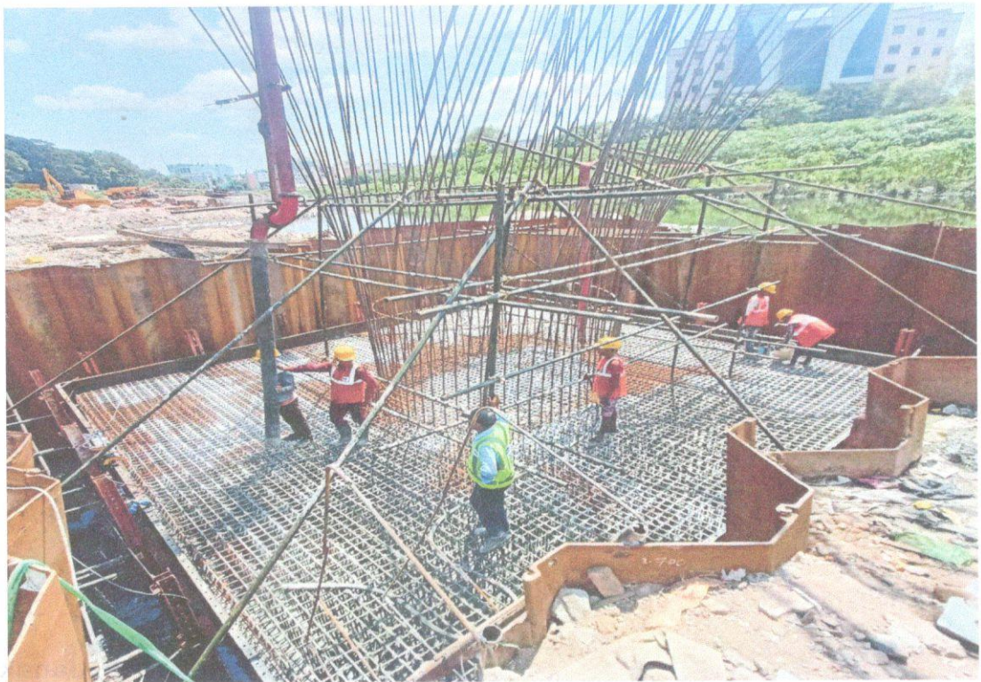
Pile cap-P 173 @ km 6+513
